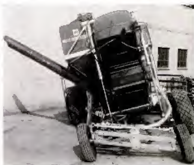
The combine can adjust for any contour. Here it is set to work down a hill that slopes to the left.
